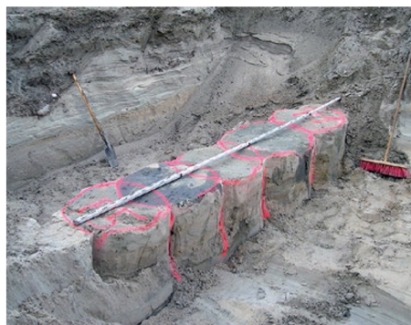
Exposed cut-off wall with Secant DSM columns
