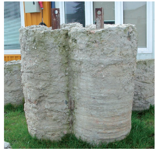
Exposed DSM columns
