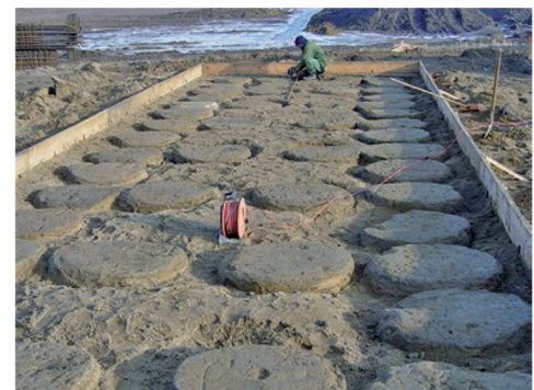
Exposed DSM columns for a bridge support
